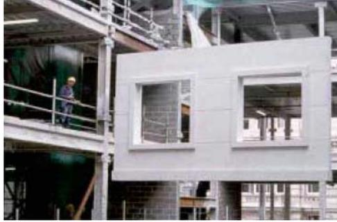
Problem: Precast panels were installed without windows. Window frames must then be installed. The work can be done from scaffolding or other methods but all involve work at height and thus a risk of falling.
