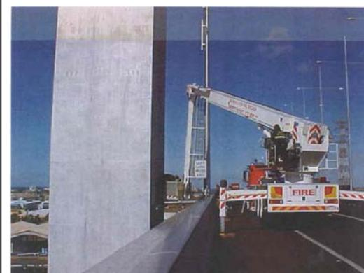
Problem: This is the Bolte Bridge in Melbourne. The two outer columns are ornamental – they are not connected to the bridge. But they need access for maintenance of the aircraft warning light at the top of the tower.
